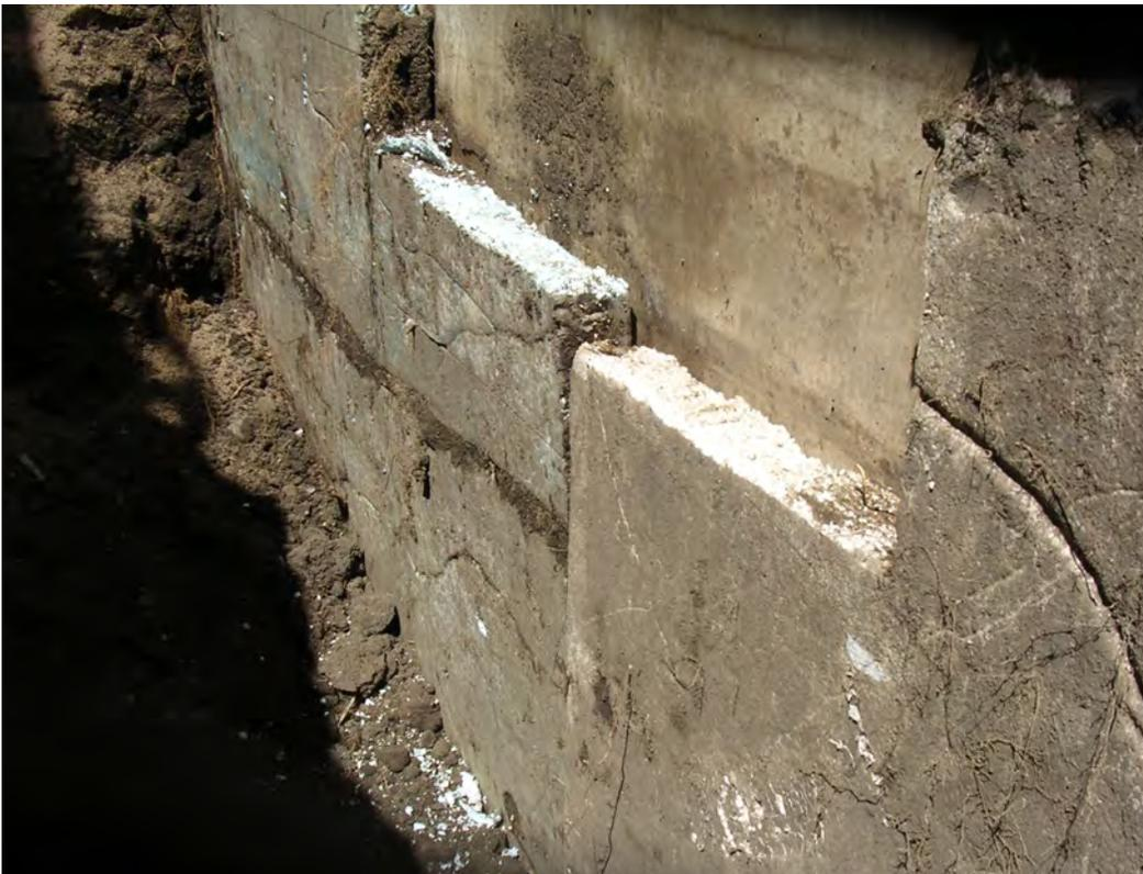
Figure 3. XPS and molded polystyrene were installed adjacent to each other
